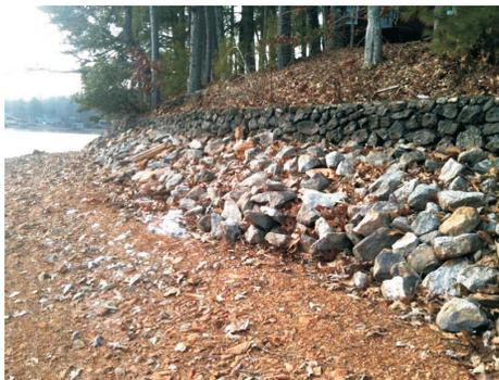
To start with, inspect the base of your seawall for exposed or undermined foundations. Any undermining should be filled (preferably with concrete). You should also inspect the grout between the stones. If it has eroded away filling these fissures with fresh grout (re-pointing) should be done to prevent further degradation. Hiring an
